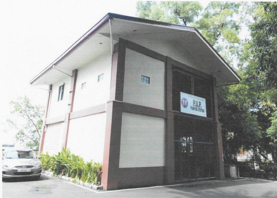
PUP PUMPING STATION
