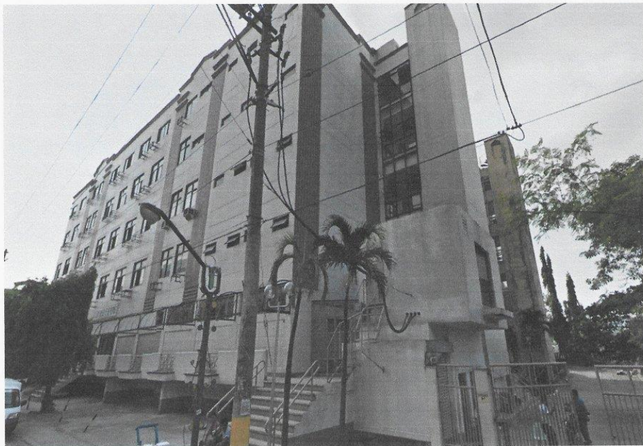
PUP CONDOTEL BUILDING
