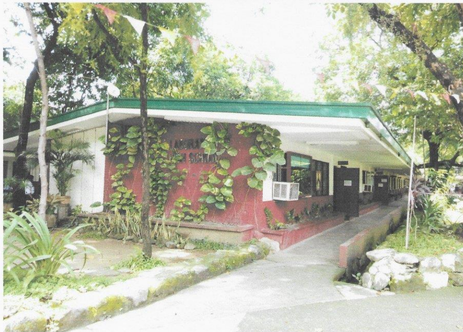
FORMER HIGH SCHOOL PREFAB
